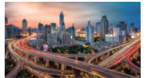
交通运输 Traffic and transportation
